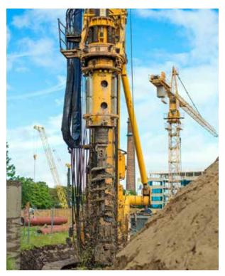
Kelly drilling is the most widespread large-hole drilling method in deep drilling technology. ZOLLERN steel profiles allow effortless transmission of torques of up to 500 kNm. The steel profiles are fitted to the so-called kelly bar, a drill pipe consisting of multiple telescopic sections, where they serve as guide and driver rails. This makes it possible to achieve drilling diameters of up to 3 metres and drilling depths of up to 90 metres.
